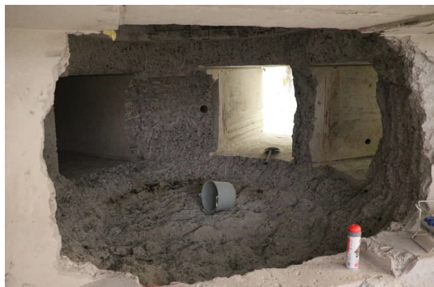
Figure 4: CAD model of the reactor biological after removing the activated concrete (left). Photo of concrete structure around two weeks before finishing the work (right).
