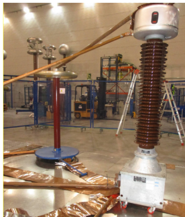
Figure 1: A HV measurement set-up for a test of an inductive voltage transformer (right) mounted at the common point. The ASEA reference divider (left).
