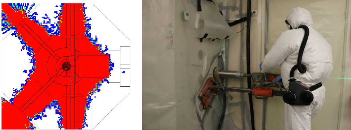
Fig 2. An estimate based on 3D inventory calculation of the activated part of the concrete in the reactor's biological shield, from which the resulting decommissioning waste is treated as nuclear waste (red). The rest of the concrete can be free released and recycled as conventional construction waste. To validate the calculation, concrete was sampled in December 2018.
